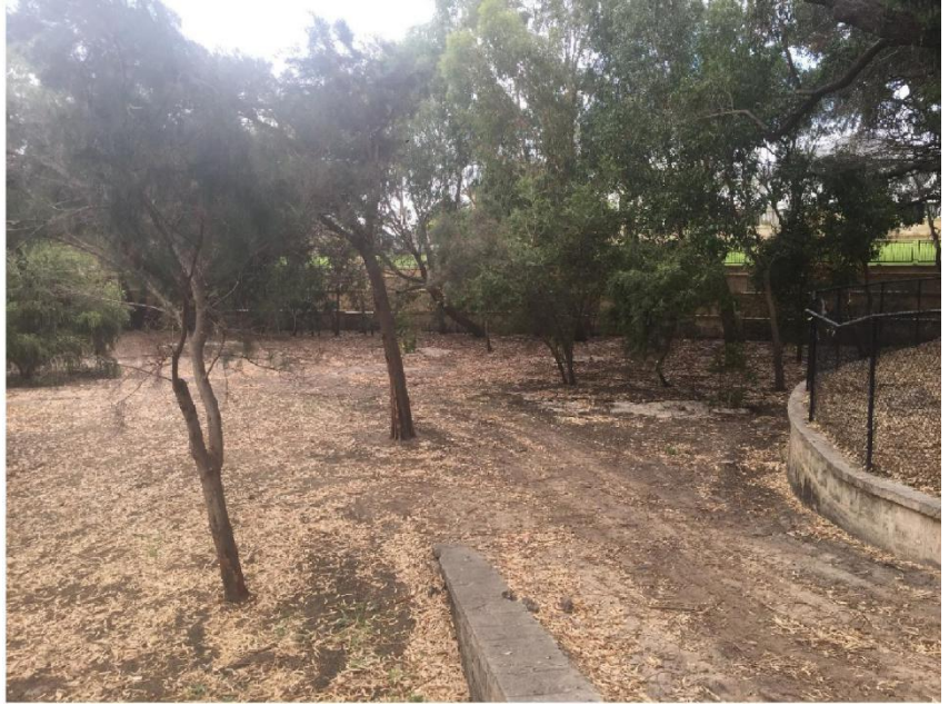
After: View into sump
