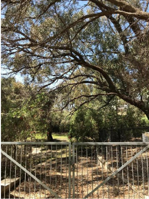
Before: View into sump
